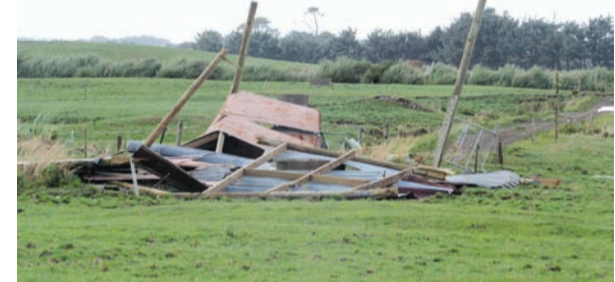
Not much left of this farm building in Kaweora Road.
