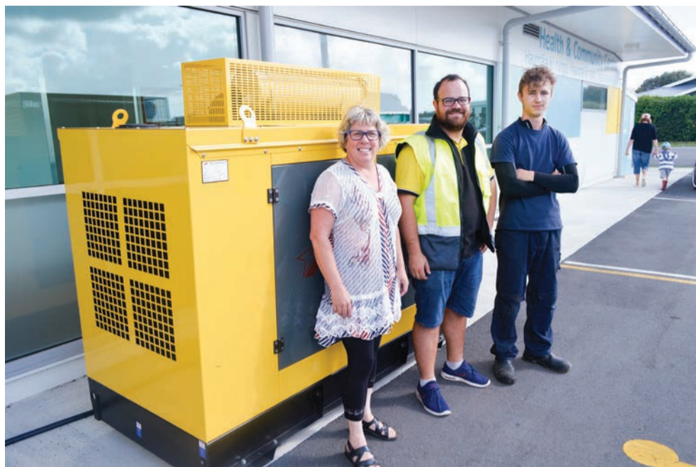
Aretha Lemon from Coastal Care with Michael Corkill and Aaron Barratt from Corkill Systems who arrived to save the day and keep the medical centre open after Cyclone Gita knocked out electricity around Taranaki with this giant generator .
